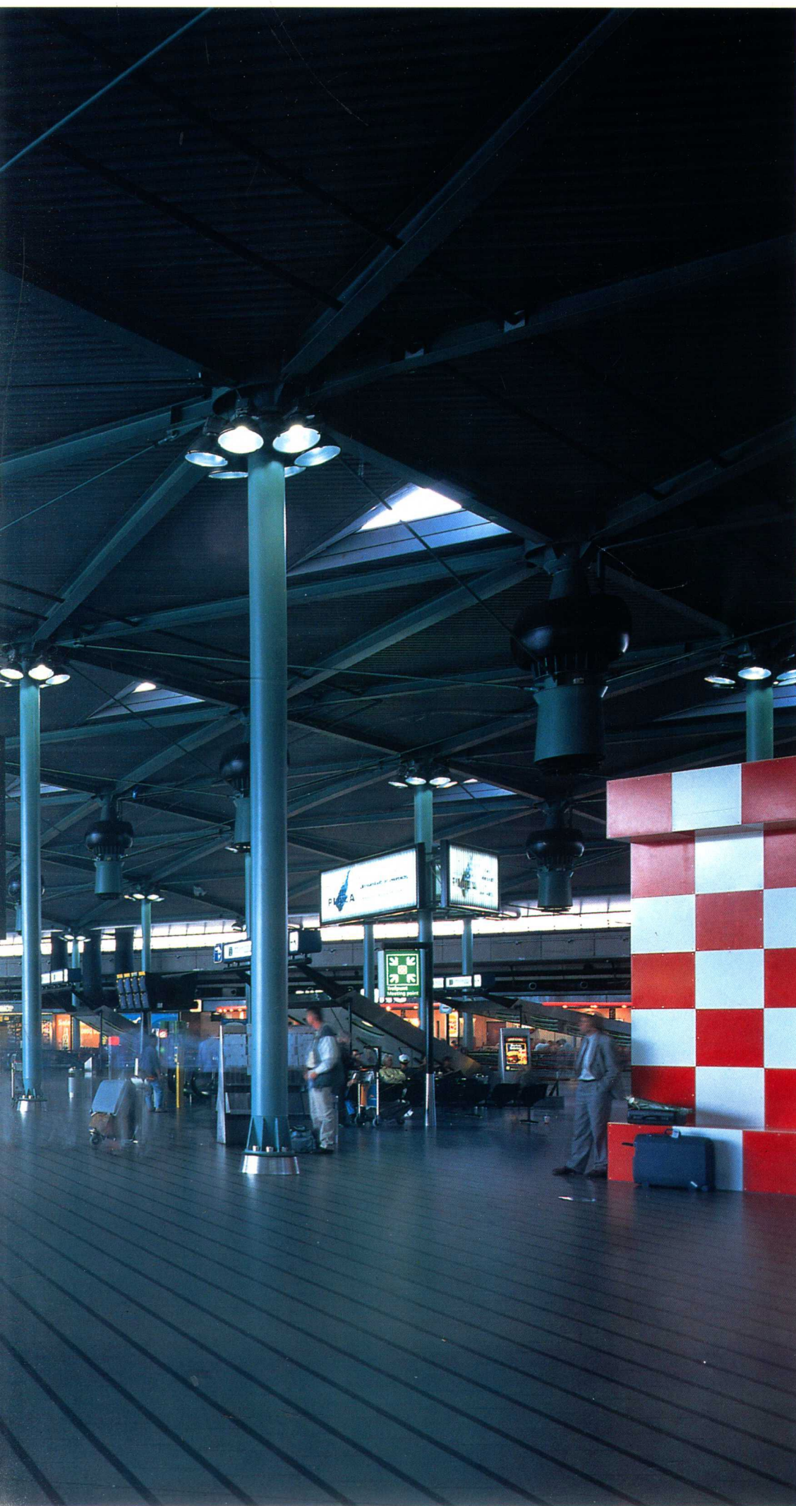
Schiphol Plaza Amsterdam Airport, Amsterdam, The Netherlands Bentham Crouwel Architekten in association with NACO, Netherlands Airport Consultants 6 Central entrance to airport Photo credit: courtesy Jannes Linders
