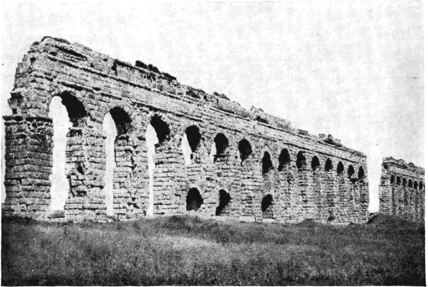
FIG. 1.—A Roman aqueduct. Claudia of dimension stone, and Novus of brick and concrete. (From " Frontinus and the Water Supply of Rome ," by Clemens Herschel.)
