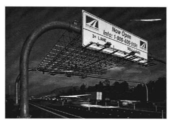
Transponders are read by overhead antennas, allowing tolls to be paid without stopping
