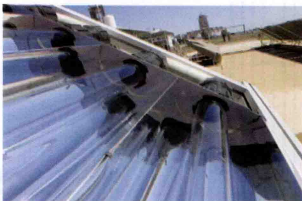
FIGURE 3.8 Photograph showing the CPC with borosilicate glass tubes (PSA, Spain).
