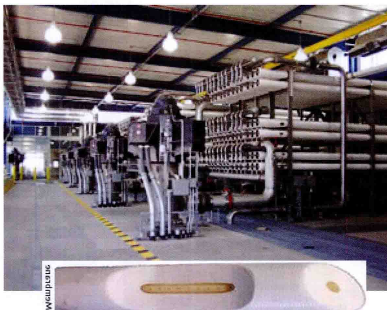
Figure 4 Membrane desalination plant. RO membrane units from El Paso Desalination Plant, Texas: the site of the world's largest inland desalination plant ( 104\,000\text{ m}^3\text{ d}^{-1} ). Production costs for water are less than less than 0.36\text{ \$ m}^{-3} . From http://www.epwu.org/167080115 .
