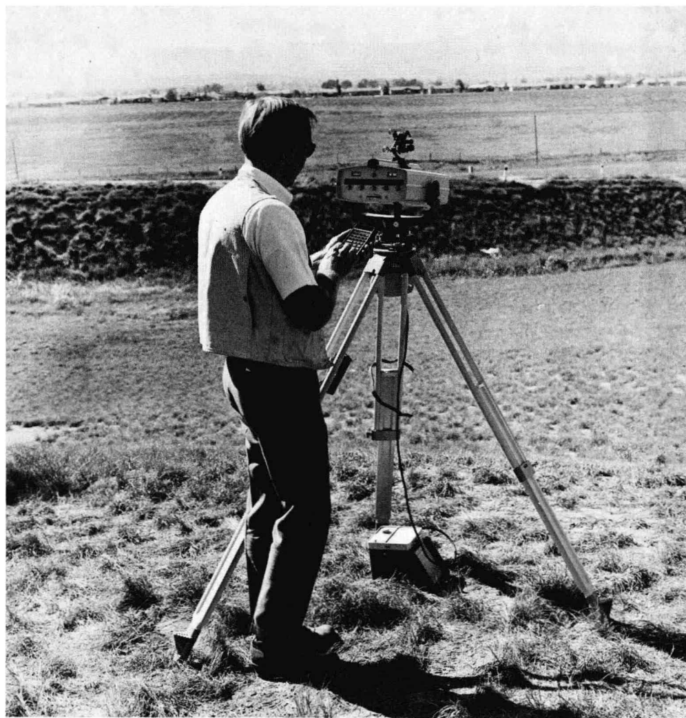
Distance meter shown in operation on construction site. (Courtesy Hewlett-Packard)
