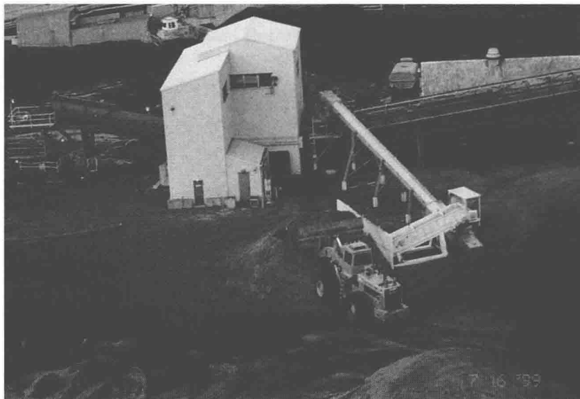
FIGURE 1.2 The on-site blending facility constructed at Bailly Generating Station for testing purposes. Note that this is a labor-intensive system. Source: [7].
