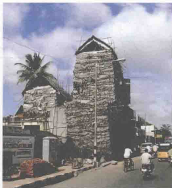
Andamiaje Construction scaffolding Pondicherry, Tamil Nadu, India
