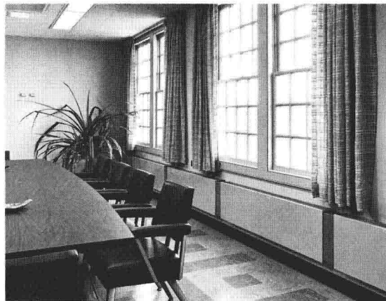
FIG. 1-5. Perimeter heat distribution by baseboard radiators. The decorative metal covers enclose hot-water (or steam) pipes to which copper or aluminum fins have been added to obtain an extended surface for maximum radiation and heat transfer to room air. (Nesbitt Div., ITT Corp.)
