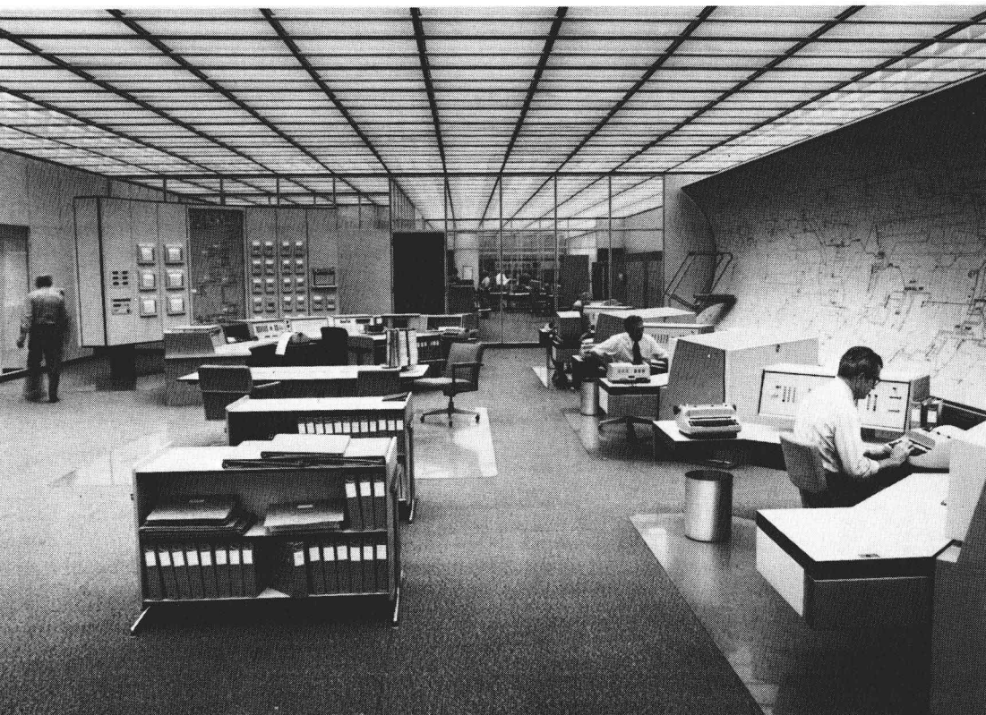
Energy control center of a large power system (Pacific Gas and Electric Company). NOTE: Control console center left with EHV dynamic board, and computer equipment in background beyond glass partition.
