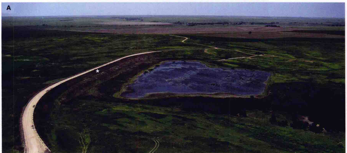
Plate 4-12A. Finney Wildlife Area in southwestern Kansas, United States. Originally designed for a much larger lake, upstream ground-water pumping has reduced spring flows, and diversion of surface water has rendered this artificial "lake" into a wetland wildlife area. During rare wet years, a tiny puddle of water is held behind this dam. Asterisk indicates position of the outlet tower. Kite airphoto by J.S. Aber.
