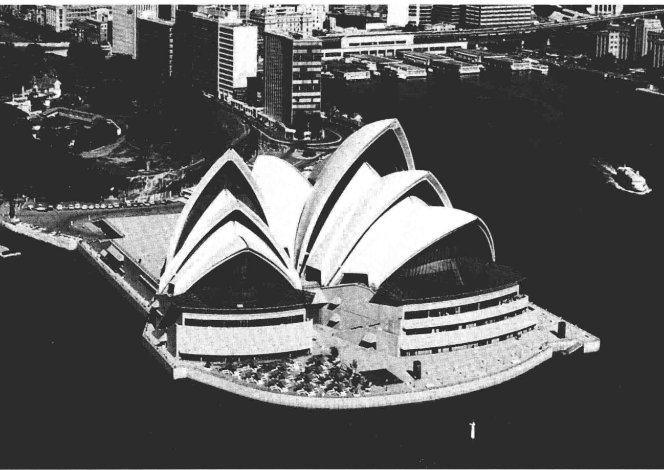
1.1 Jorn Utzon and Ove Arup: Opera House, Sydney, 1973. (photo: WGBH/ Nova)
