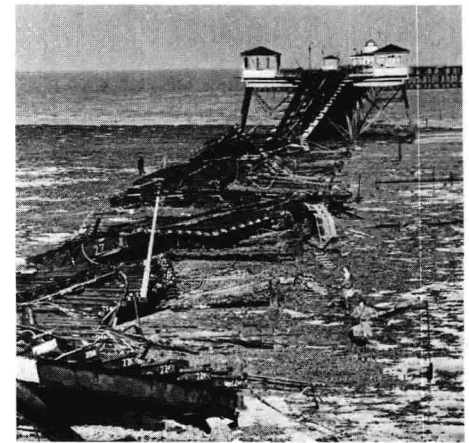
Figure 1.3 A damaged pier
