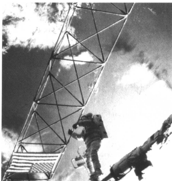
Figure 2. NASA photograph showing an astronaut constructing a boom in space
