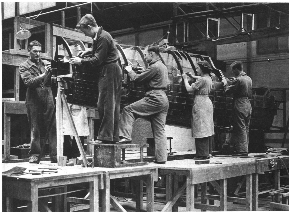
Fig. 1.4 The Spitfire fuselage designed and built of Gordon Aerolite material by Aero Research Ltd, Duxford in 1940. Metal was used only in the mainspar members and certain pick-up fittings. Aerolite was composed of untwisted flax fibres impregnated with phenolic resin and made into 6 in wide bands. To produce sheet material the bands were placed edge to edge on moulds with others at right angles to build up thickness. The pack was then hot pressed. Ciba-Geigy Plastics
