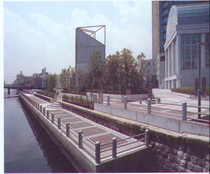
Water embankment at Sibaura Canal side 芝浦運河側の親水護岸
