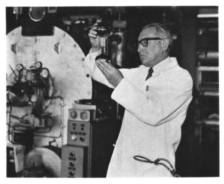
I/5 Periodic checks of combustion plant performance can be carried out fairly easily using simple indicators to measure the carbon dioxide content of the flue gases, and by measuring temperatures and smoke levels. All the instruments required can be included in a small portable test kit.
