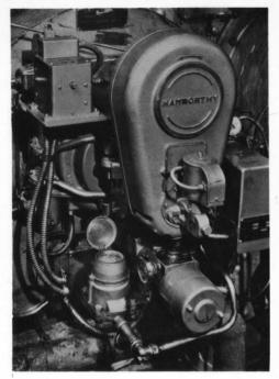
1/3 Simple measurement of energy input to individual major items of plant is invaluable for control purposes. A small, positive-displacement oil meter fitted to the oil supply line to burners on a steam boiler.
