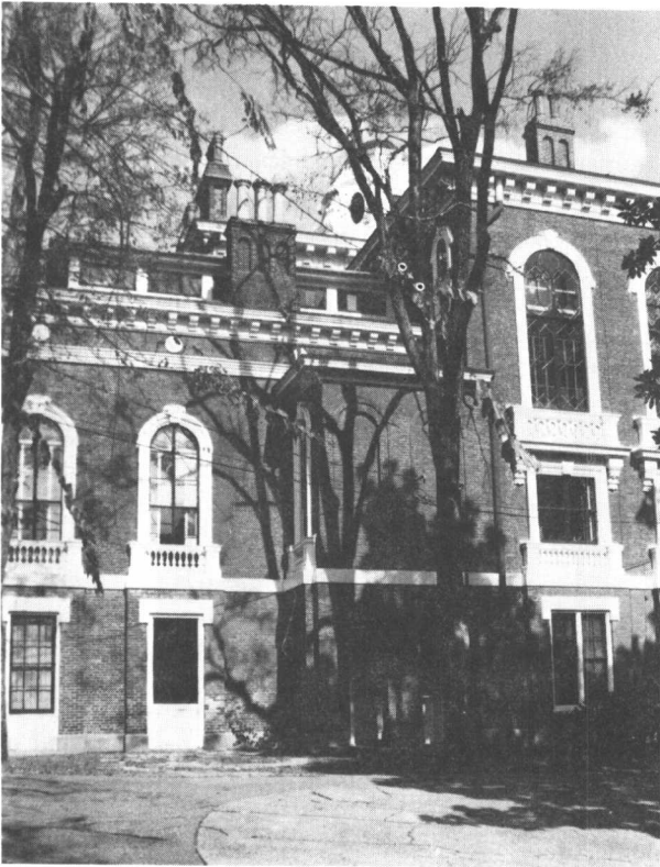
Figure 1.2. Hay House, rear elevation.
