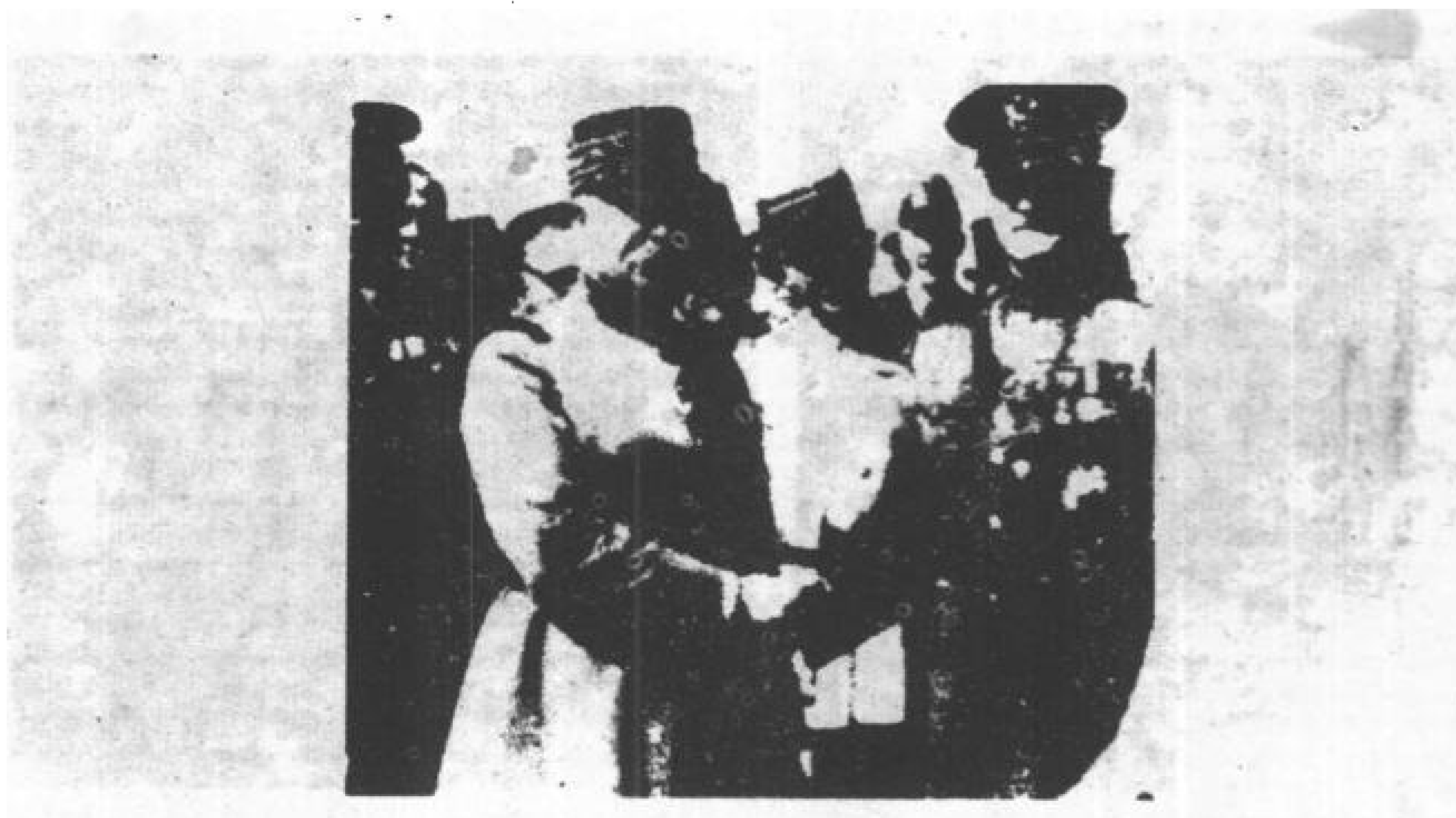
Figure 1.3. Unretouched cable picture of Generals Pershing and Foch, transmitted by 15-tone equipment from London to New York. (From McFarlane [1972].)
