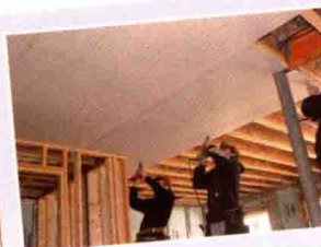
FIGURE 17-40 This photo is of the same drywall piece being installed as in figure 17-39. It is now obvious why such a steep angle was necessary. This size and cut of drywall is a challenge to install that is solved by using teamwork.
