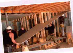
FIGURE 17-39 Workers are installing drywall that is 16 feet long. Sheet is at a steep angle and looks improper, but it was done to make it fit into a cut provided for the post.
