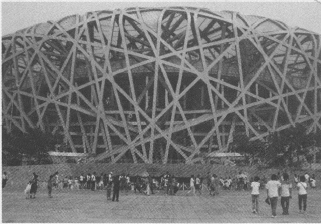
Fig. 7 The "Bird Nest" for 2008 Olympic Game was made of HSLA steels, Q420 and Q460
