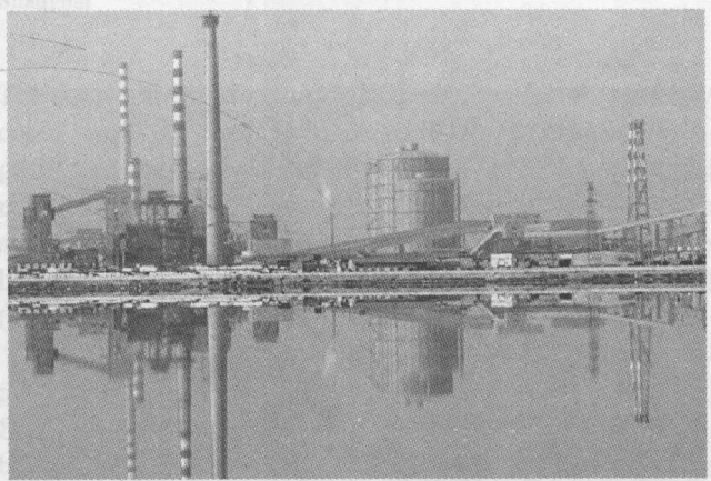
Fig. 6 Caifeidian, a newly constructed steel plant in China, possesses three fundamental roles: steel production, energy conversion, and waste treatment
