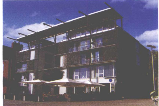
PV shading device integrated into the building design
