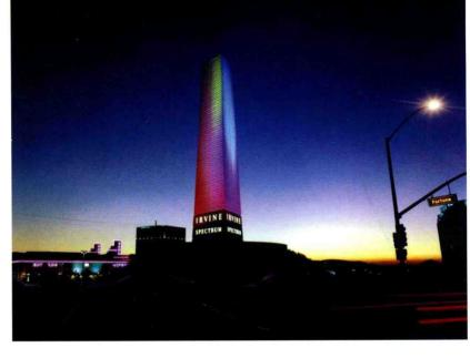
This 90-ft. tower is fabricated from galvanized steel supports and light-absorbing fiberglass panels. The lower ID aluminum panels are routed and have filled-in letters. At the tower base, 21 independent spotlights are computer-driven to change multi-colors and intermittently illuminate the tower. The tower also houses Airtouch Cellular's full antenna array for all of Southern California and surrounding areas.
