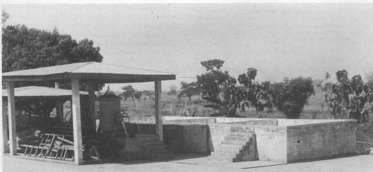
Figure 3.5. Parboiling plant in Ghana equipped with concrete soaking tanks and tip-over steaming pans
