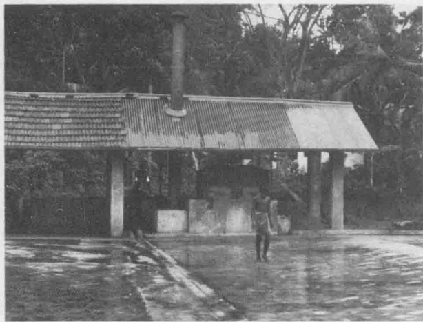
Figure 2.3. A primitive parboiling plant in India: the drying floor is in the foreground
