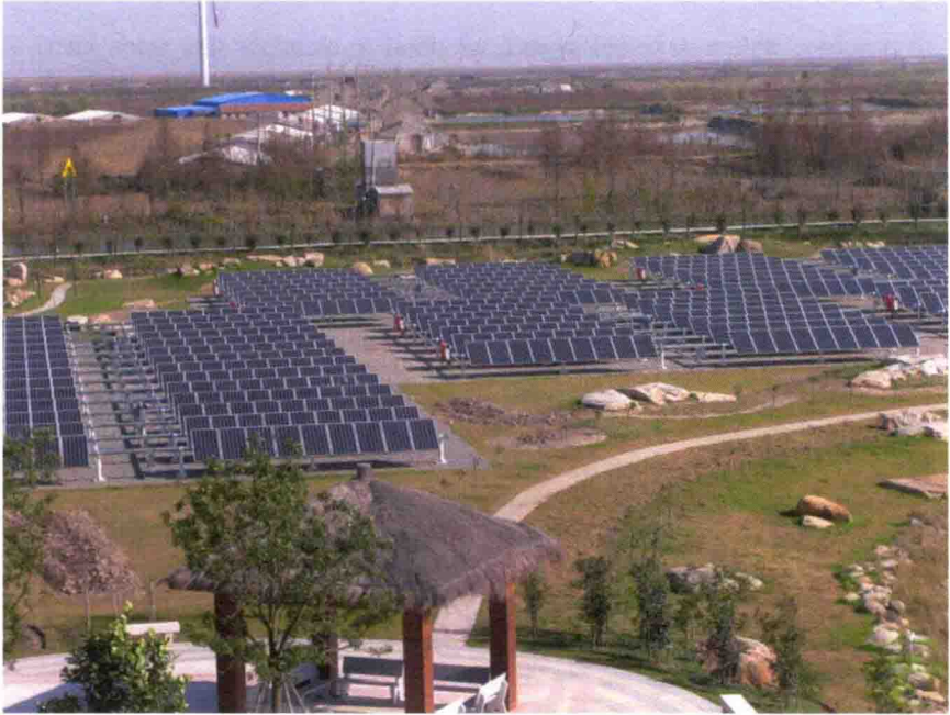
This photograph shows a 300 kW solar cell field near Shanghai China designed and installed by the authors company in 2008. The largest solar field in operation at the end of 2013 is one thousand times larger at 300 MW. In 2018, there will be multiple GW sized solar fields in operation around the world
