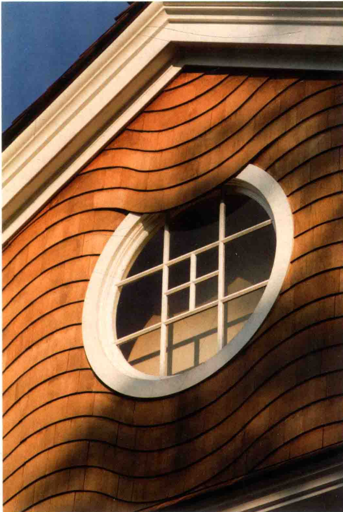
Left: High-performance windows and cedar shingles combine character with environmental consciousness.
