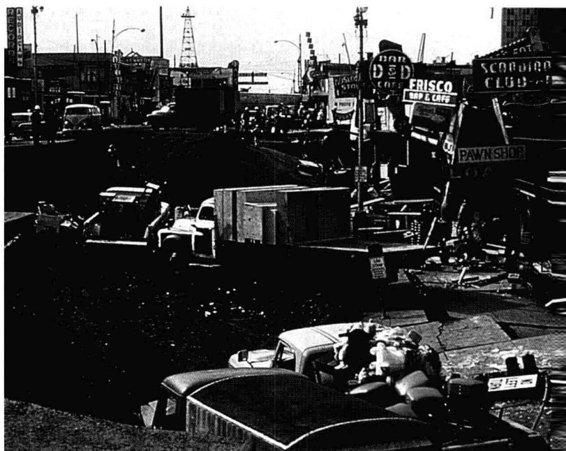
FIGURE 1.2 Fourth Avenue, Anchorage, Alaska, after the 1964 earthquake. Note how far the shops and street on the right have dropped relative to the left side of the street.
