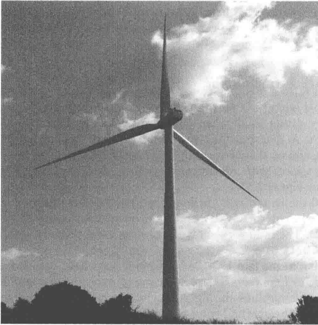
Figure 1.2 Gamesa G128 with 4.5 MW nominal power, 120 metre hub height and 128 metre rotor diameter is a new large wind turbine from the Spanish manufacturer Gamesa (photo: Tore Wizelius)
