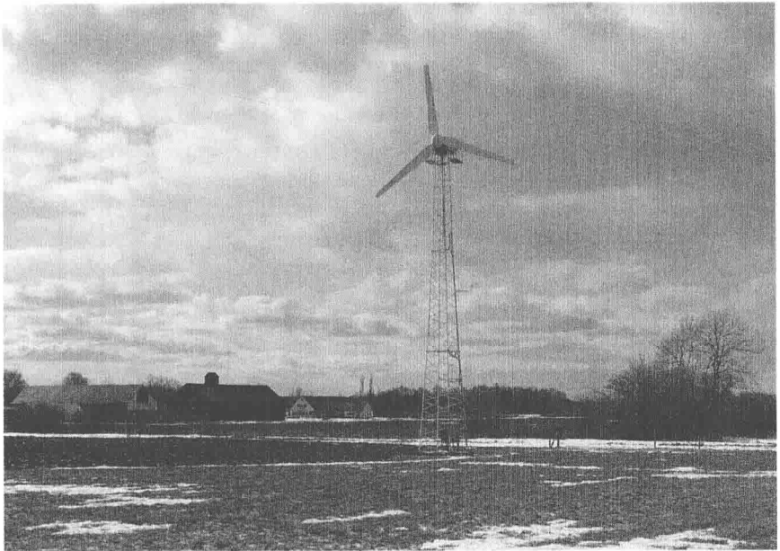
Figure 1.1 Typical wind turbine from early 1980s. A Vestas V15 with 35 kW nominal power and 18 m hub height installed at Lövsta Agricultural School on Gotland (photo: Tore Wizelius)
