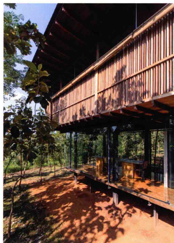
Top: Openable shutters and minimal glass promote cross-ventilation in the Channa Daswatte House.
