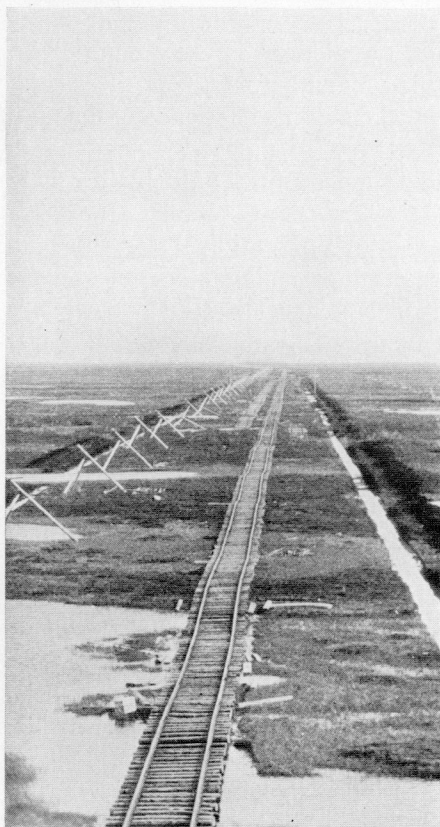
FIG. 3—Telephone line on temporary tripods and new track in undeveloped country, Hudson Bay Railway. (Canadian National Railways.)
