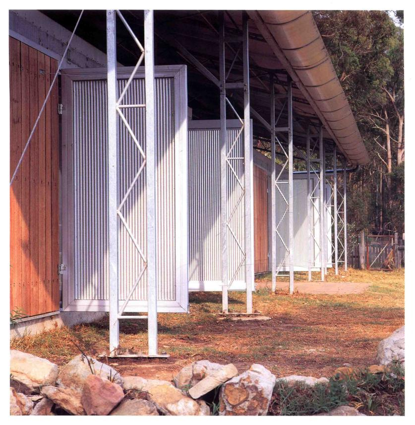
The double covering allows for ventilation of the interior living spaces and regulates temperature and lighting. Water is collected in large tanks that can provide water reserves for many months.
