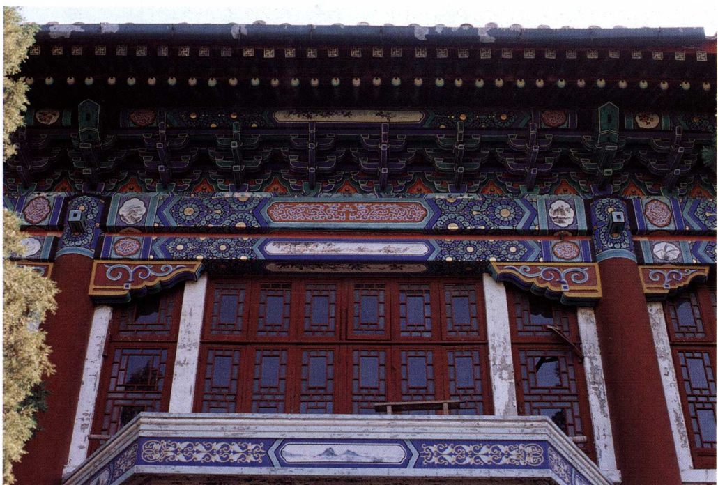
Plates 4 and 5 Eaves, cornices and other elevation details of buildings at Beijing University, designed by Henry K. Murphy in the mid-1920s.
