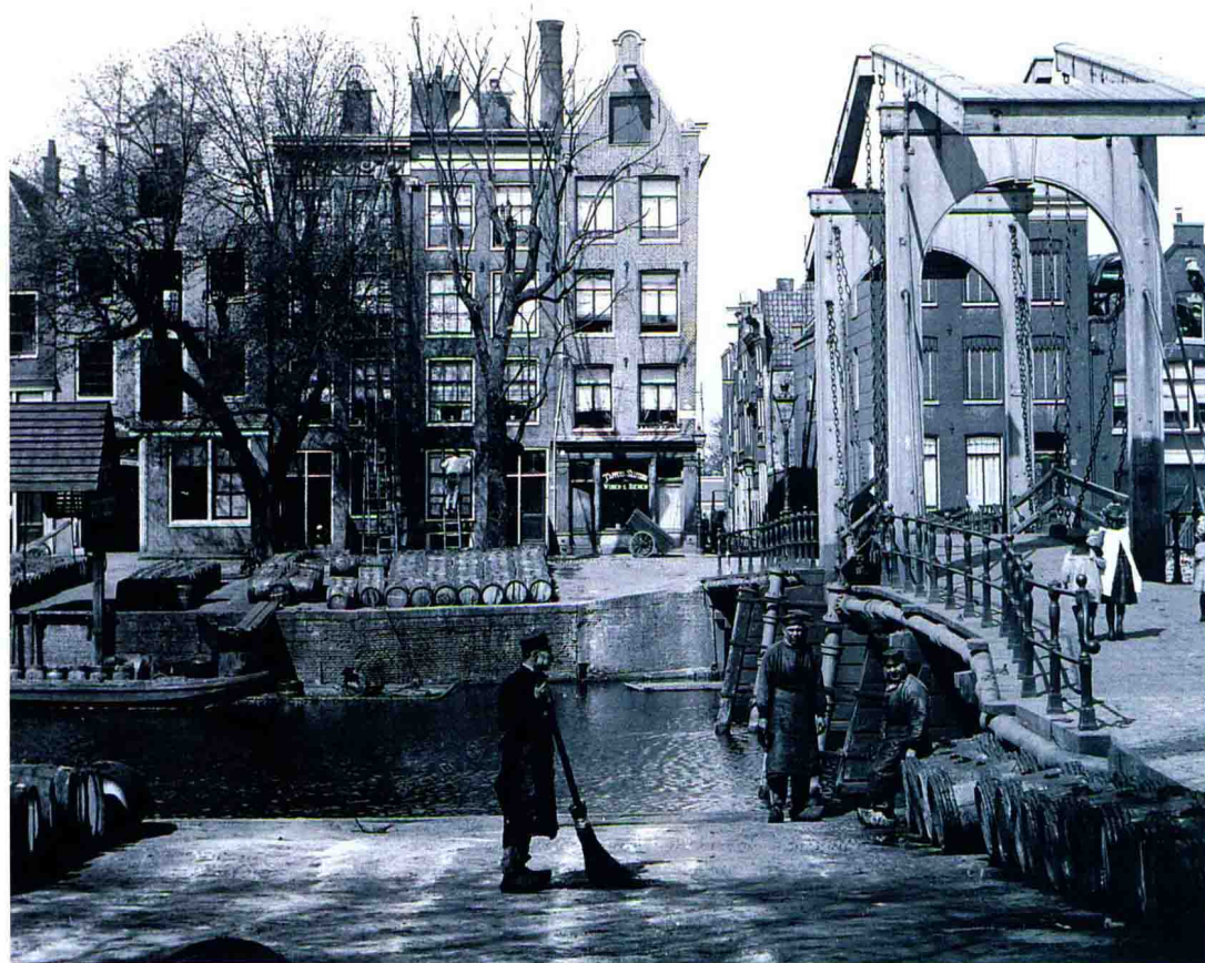
Nieuwe Teertuinen 19 to 15 (r. to l.) Looking towards bridge no. 321 ('Sloterdijkbrug') and the start of Sloterdijkstraat. Left is the 'de Roosos' tar company with a hoist to lift the barrels of tar out of the barges on the canal (the last windlass in Amsterdam). Photo Olie Jansz, Jacob (1834-1905)
