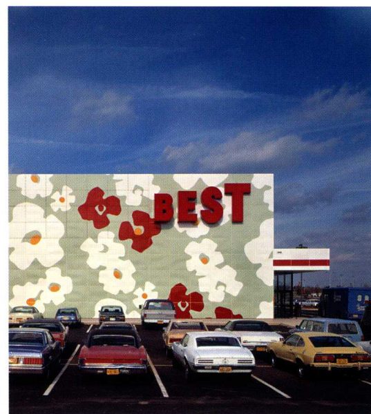
BEST Catalog Showroom, VSBA, Langhorne, 1978 Robert Venturi and Denise Scott Brown dressed up an otherwise banal box with their signature oversized graphics in a design for a BEST Products Catalog Showroom in Pennsylvania.
