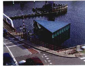
17. Bridgehouse BAR architecten Middelburg, 2004
