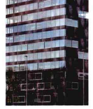
80. The V Tower Wiel Arets Eindhoven, 2009
