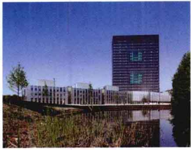
56. Westraven Cepezed Architects Utrecht, 2007
