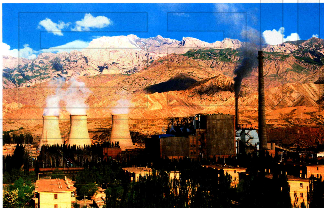
拜城火电厂 Baicheng thermal power Plant
