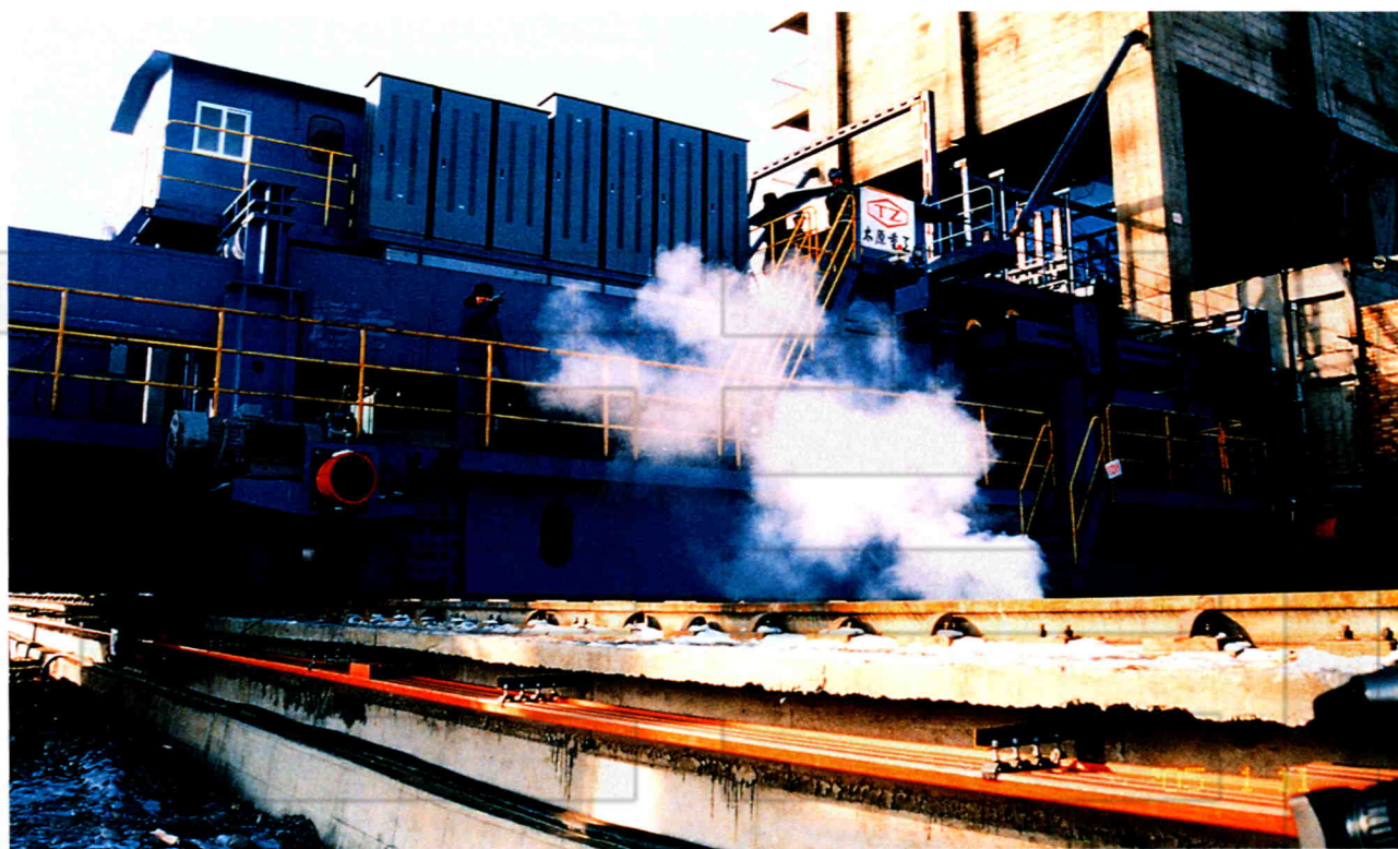
拜城百万吨煤焦化厂 Baicheng Coal Coking Plant with annual output of a million tons
