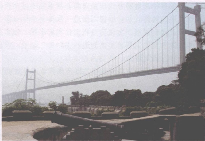
▲虎门威远炮台，远处为虎门大桥
