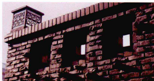
图13 疙瘩砖细部 Fig.13 Detail of bricks with coarse and lump surface
