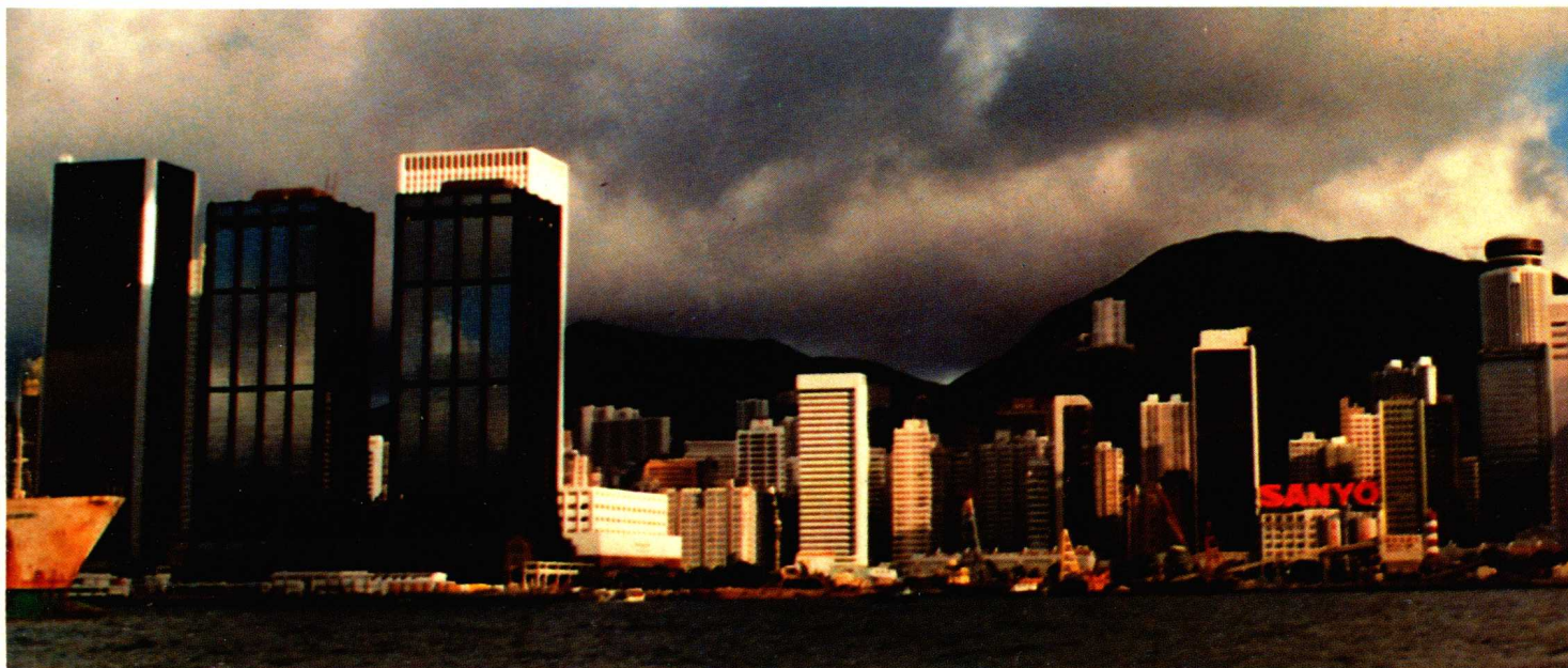
Wan Chai Harbour Building View 灣仔海傍建築羣
