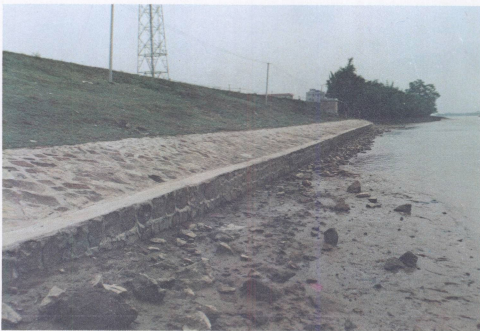
挂影洲围北堤砌石护岸
