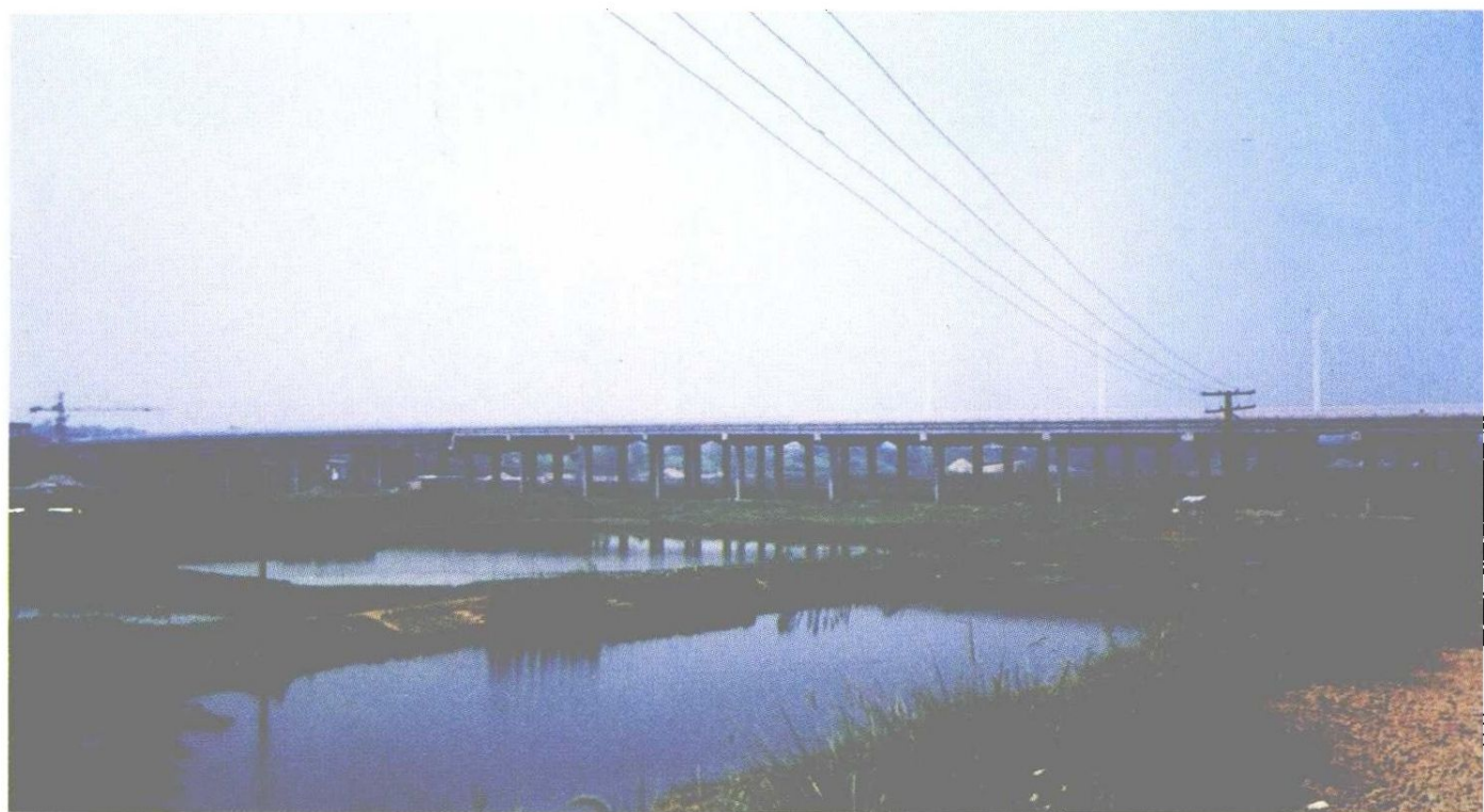
▶ 境内市外环路蒸水桥
