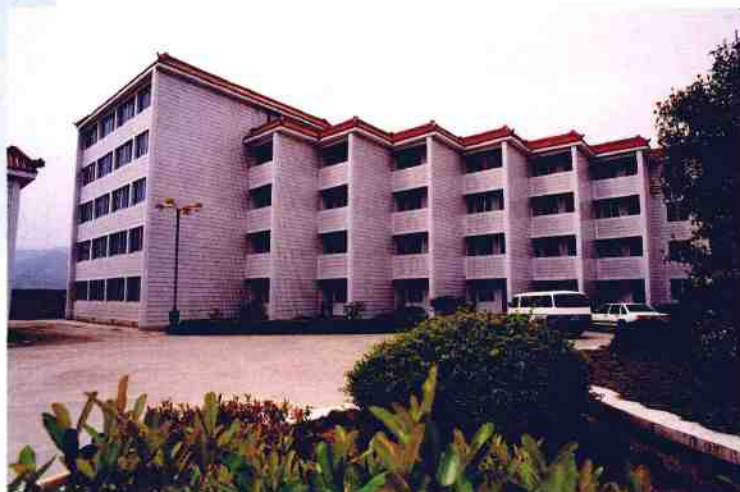
公用事业楼 The public administration building
