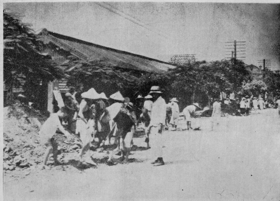
Repairing Highway Near Tai-Chung
