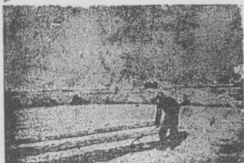
Fig. 3. Spreading feces on drying field. Feces cakes in Storage in background.
