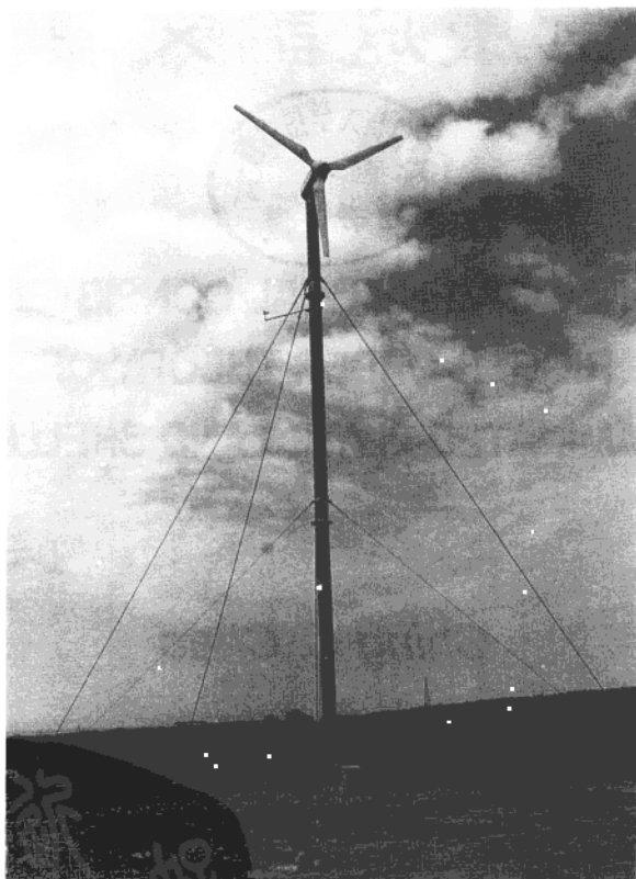
3 kilowatt glass/epoxy form sandwich wind turbine blades of 3 meters long - design, analysis and prototype manufacturing - an Energy Resources Research Project supervised by Professor C. C. Chao, Hsinchu, Taiwan, R.O.C. 1982.
