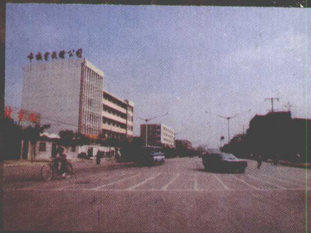
新建的工業路 Newly built Industrial Road
