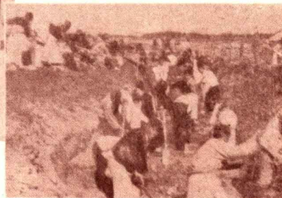
Soochow inhabitants serving to dig trenches.
