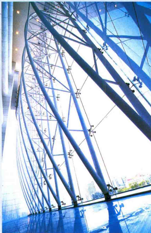
弧型桁架点式玻璃幕墙 Glass Curtain Wall Of Arc Girder Spot
