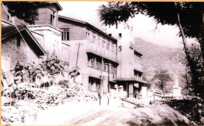
东北大学在本溪 The Campus of the Northeast University in Benxi
