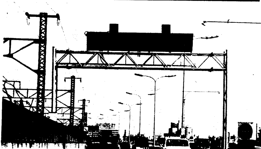
Figure 7. Variable information indication device and ultra sonic detector along expressway.
